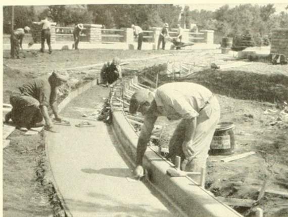
WPA workers have built thousands of miles of curbs and gutters and many other highway improvements
