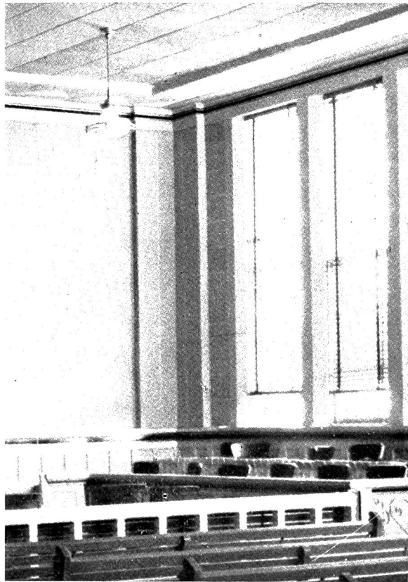
MAJOR ALTERATIONS MADE TO COUNTY COURT ROOM INCLUDED LOWERING THE CEILING AND COVERING WALLS WITH SOUND-ABSORBING BOARD
