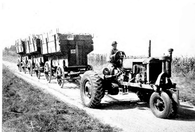
International Harvester Co. THIS TRACTOR EQUIPPED WITH PNEUMATIC TIRES REPLACES THREE DRIVERS AND TEAMS AND DOES THE WORK MORE QUICKLY
