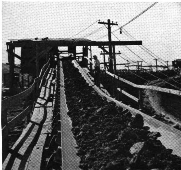
BELT CONVEYOR REMOVING EXCAVATED MATERIAL
