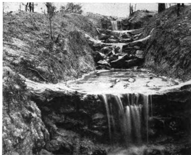
ROCK DAMS TO CHECK GULLY EROSION
