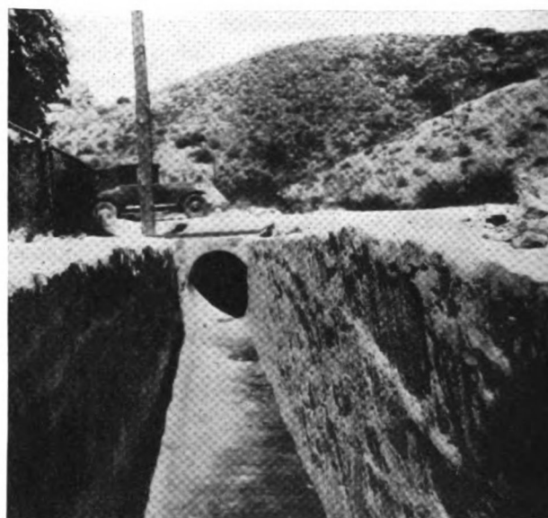
SECTION OF A W. P. A. FLOOD CONTROL DRAIN
