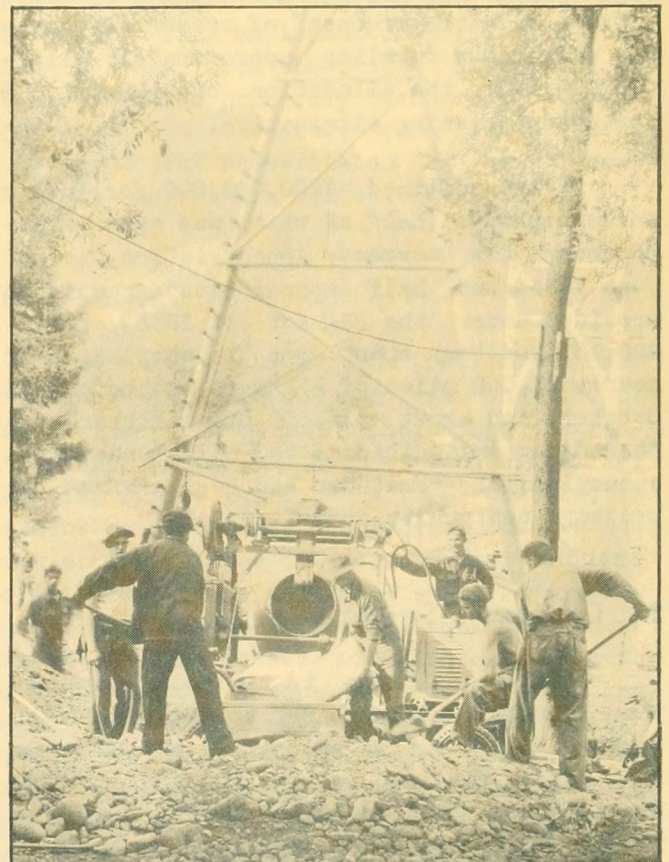
MIXING CONCRETE FOR A CCC BRIDGE
