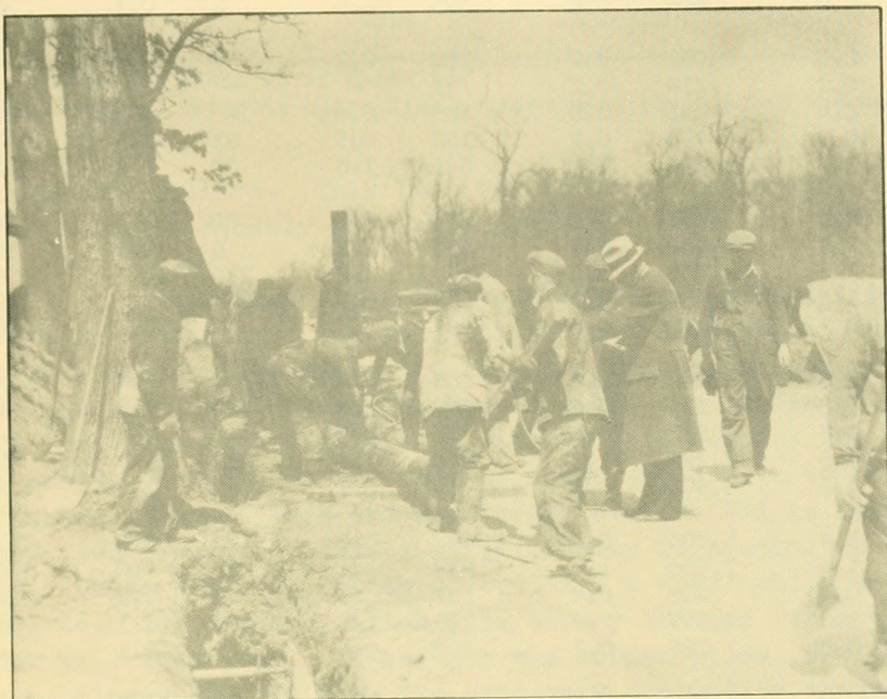
WPA WORKERS ROLLING A MAIN INTO PLACE FOR A WATER SYSTEM
