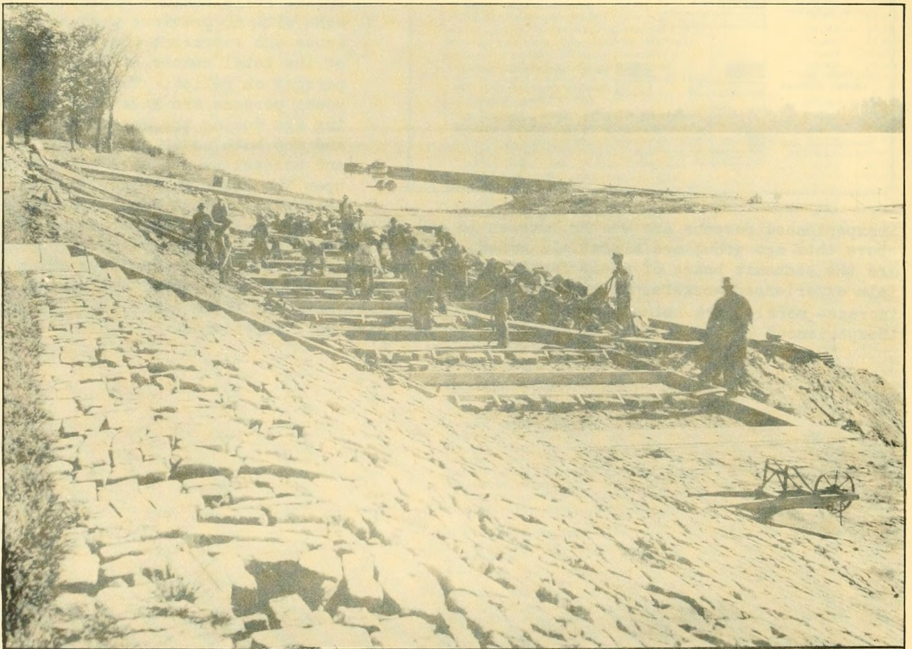
CONSTRUCTING FORMS FOR CONCRETE PAVING TO IMPROVE A RIVERSIDE ESPLANADE
