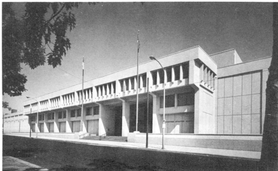
Exterior view of the new United States Mint facing Fifth Street, Independence Mall, Philadelphia, Pennsylvania.
