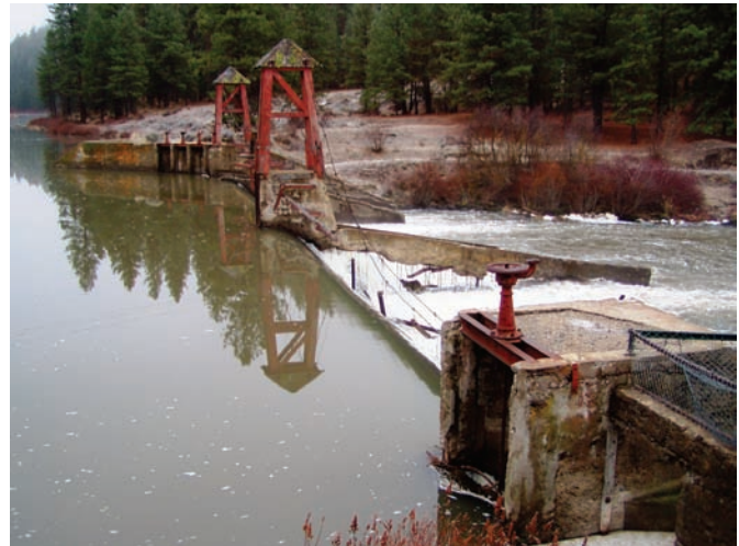
Removing the aging and dilapidated Chiloquin Dam will open up many miles of spawning habitat to endangered fish. Installing pumps will allow irrigators to continue to get the water once provided by the dam.
