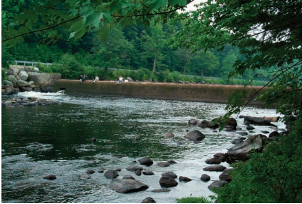
The Henniker dam in New Hampshire before removal.
