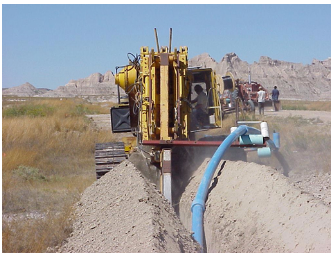
There are 10 more like it. Eleven different Federal programs help rural communities build water infrastructure.
