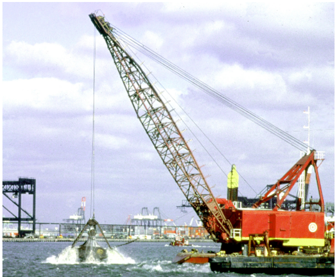
A top bottom. The Budget provides $103 million to dredge and improve the Port of New York and New Jersey. This is one of eight top priority projects identified in the Budget. The estimated net benefits of the construction under way are two times greater than the costs.
