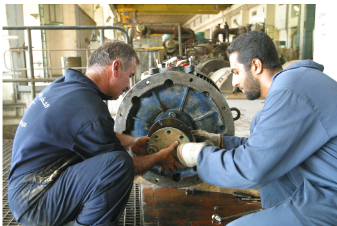
Working to restore electricity.
