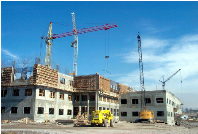
Ongoing embassy construction in Yerevan, Armenia.
