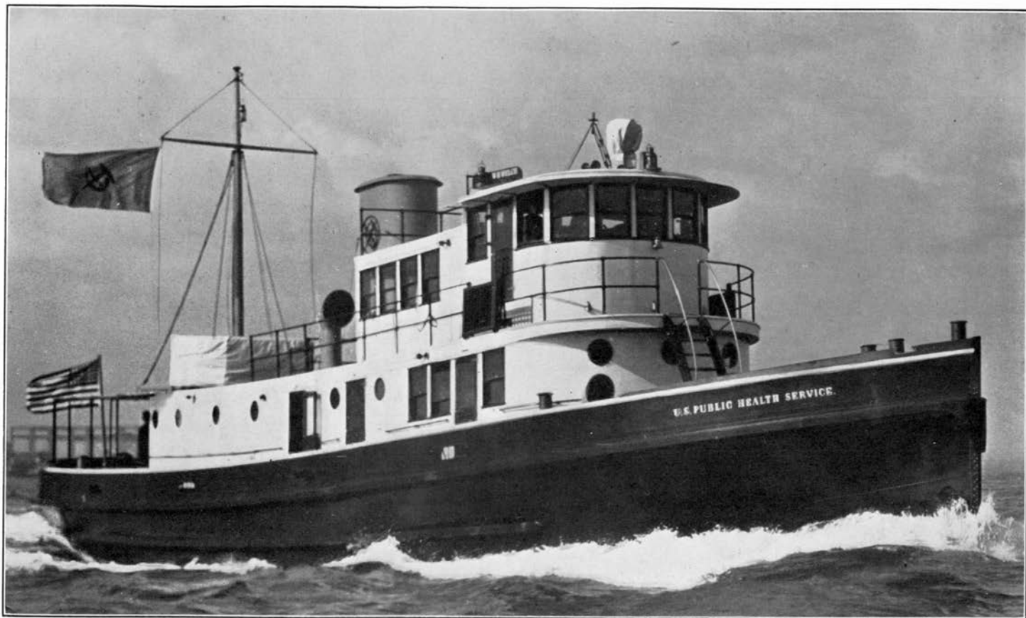
THE QUARANTINE LAUNCH "W. H. WELCH", A 100-FOOT BOAT DESIGNED FOR INSPECTION AND FUMIGATION WORK AT THE LARGER PORTS.
