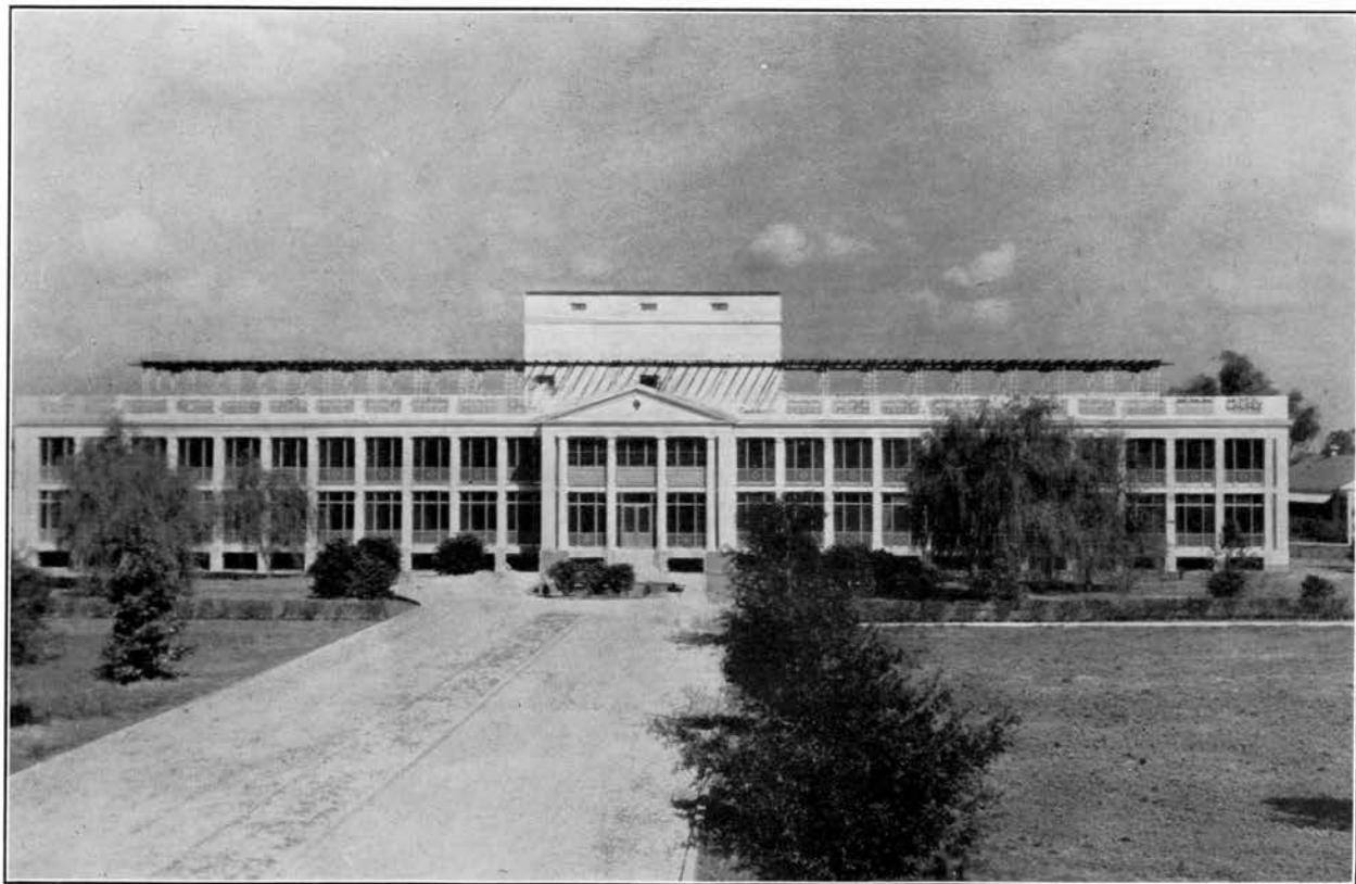
NEW INFIRMARY BUILDING AT THE NATIONAL LEPROSARIUM, CARVILLE, LA.
