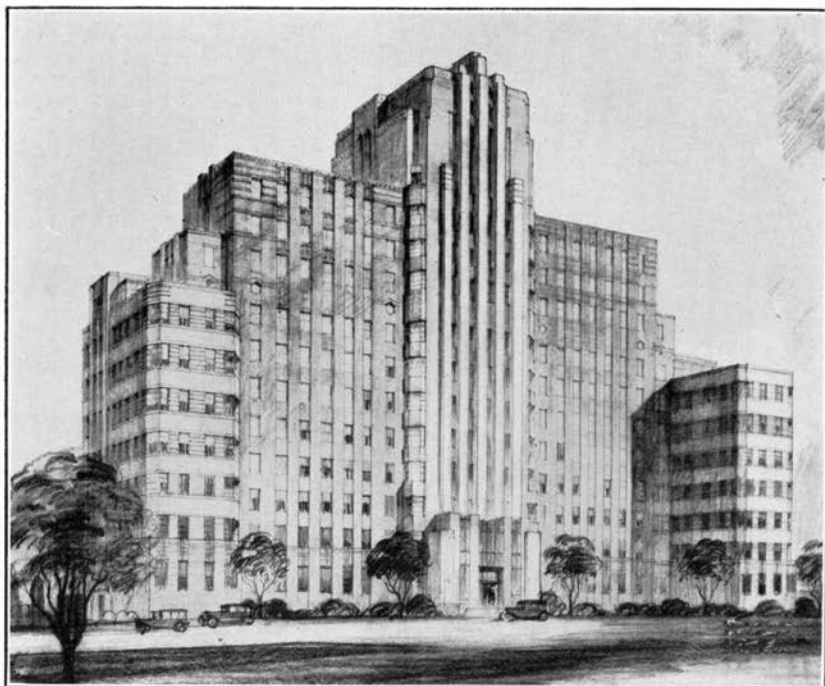
UNITED STATES MARINE HOSPITAL, SEATTLE, WASH., TO BE COMPLETED IN 1932
