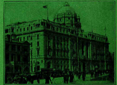
Hongkong and Shanghai Banking Corporation, Shanghai, China
