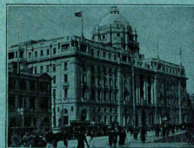
Hongkong and Shanghai Banking Corporation, Shanghai, China
