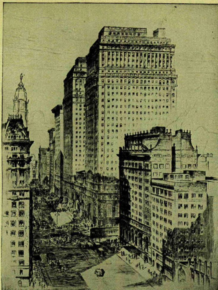
South Broad Street Looking North
