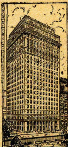
Company's Home Office Building
