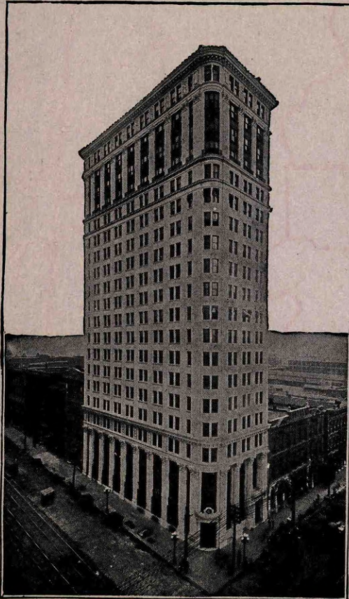
American Trust & Savings Bank Building
