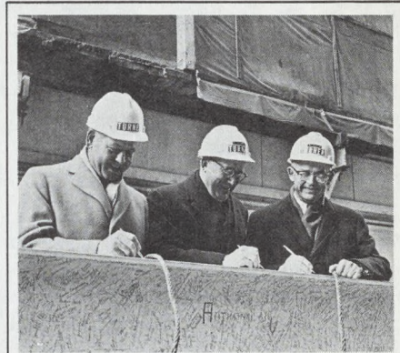
PICTURE OF THE WEEK — Top officers of Chicago's Northern Trust Bank added their signatures to the topping out beam of the 31-story Northern Building at recent topping out ceremonies. Chairman of the board Edward Byron Smith (center), President E. Norman Staub (left), and Vice Chairman Douglas R. Fuller joined more than 2,000 employees and customers who signed the beam during its two-week display in the bank. The Northern Building will be completed in 1974 at the northeast corner of Wacker and Adams in Chicago's Loop.
