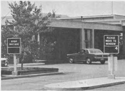
Two electronic control panels "direct" drive-up traffic at First National Bank, Mattoon, Ill.
