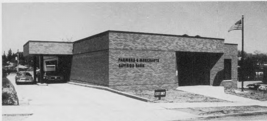
The new Farmers and Merchants Savings Bank in Waukon features a double drive-up teller, along with a new ATM system for customer convenience. Executive Vice President Ed Lauerman notes that the ATM is especially popular with older customers.
