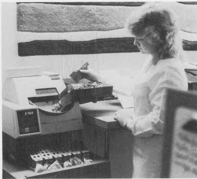
LOCATED in the vault at Sheridan Bank, Peoria, Ill., is the Brandt Model 855 Cash Settlement System. Here, currency totals processed on the Model 872 Currency Counter are transmitted to the Model 855 Central Control Unit.
