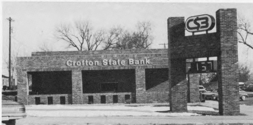
CROFTON State Bank officially opened its doors in its new building earlier this year with an open house. The new facility is located on the corner of Second and Kansas Streets and is the former Crofton Feed and Implement building. Tours were given of the remodeled facility along with drawings held for prizes and gift certificates.
