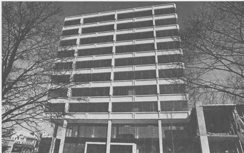
First National Bank of Des Plaines
