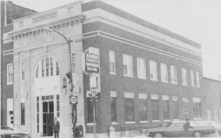
PICTURED is the newly-remodeled Hardin County Savings Bank, Eldora. The building was extended north to an alley with the addition including a new vault, conference room, private offices, consumer loan department and insurance agency. The former vault was torn out to make room for four new offices and the farm management department. R. R. Brown is the bank's president.
