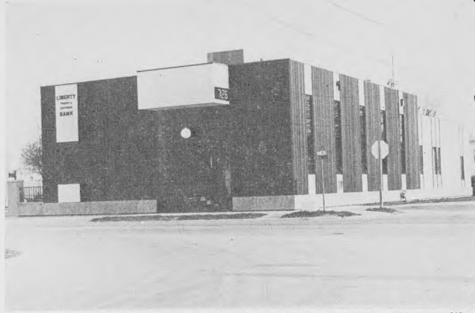
SHOWN above is the Liberty Trust & Savings Bank, Durant, before and after remodeling. The original structure had a high ceiling and a second floor was added without changing the roof structure by using I beams. The bookkeeping department is now located on the second floor with a balcony overlooking the lobby.
