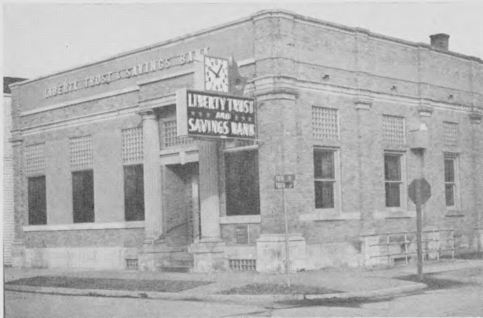
SHOWN above is the Liberty Trust & Savings Bank, Durant, before and after remodeling. The original structure had a high ceiling and a second floor was added without changing the roof structure by using I beams. The bookkeeping department is now located on the second floor with a balcony overlooking the lobby.
