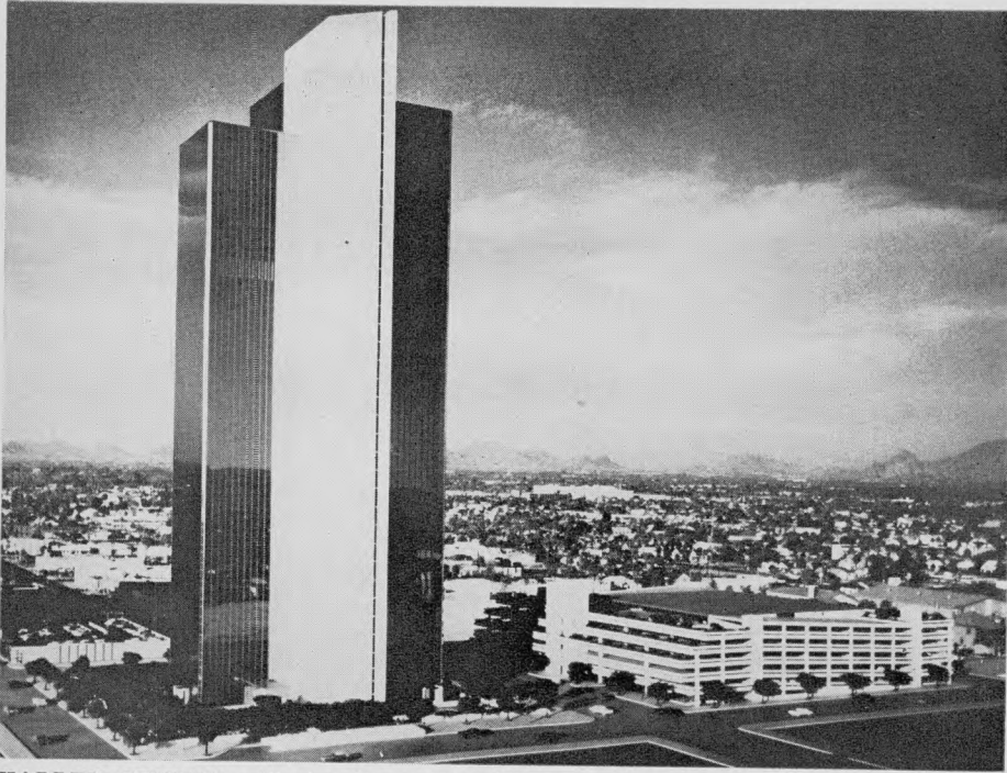
VALLEY CENTER will rise 35 stories high and will be the tallest building in the Southwest. This composite picture shows the model of the Valley National's new home office building and parking facility (right) superimposed against Phoenix skyline.
