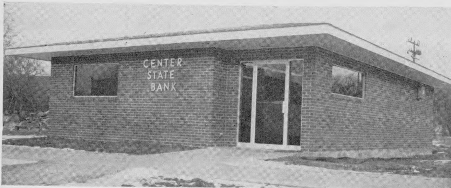
NEW BUILDING for Center State Bank at Center, Nebr.
