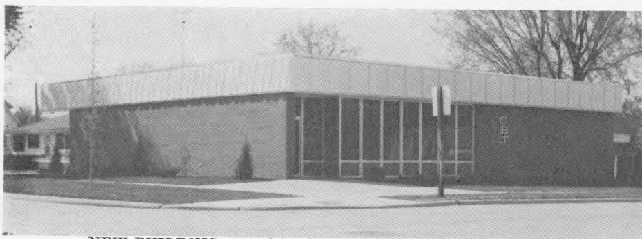
NEW BUILDING opened by Community Bank & Trust in Traer.
