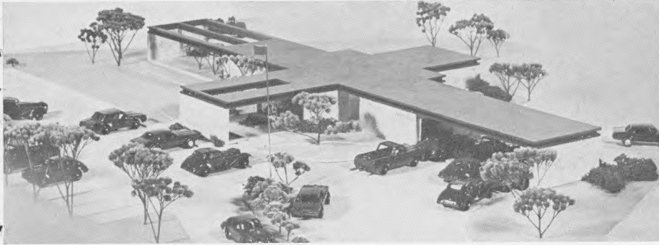
NEW FACILITY for First Natl., Dubuque.
