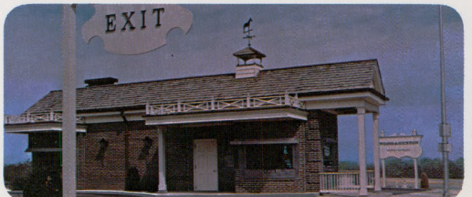
5 Wood & Huston Bank, Marshall, Mo.
