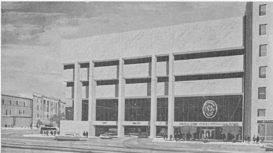
SOUTH SIDE of U. S. Natl. Bk. of Omaha's new bank building. Farnam St. is in foreground; 20th St. at left.
