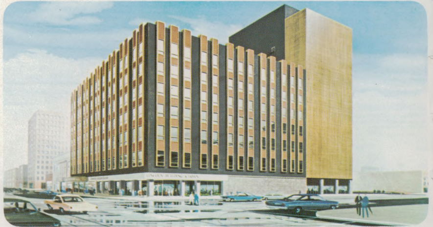
2 Lincoln Federal Savings & Loan, Louisville, Ky., after.
