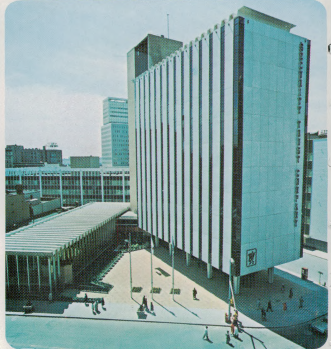
3 Multi-story Security Trust Company, Rochester, N. Y.
