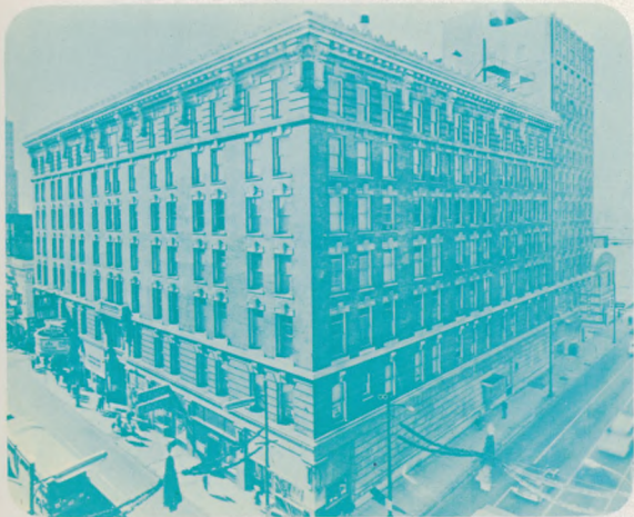
1 Lincoln Federal Savings & Loan, Louisville, Ky., before.
