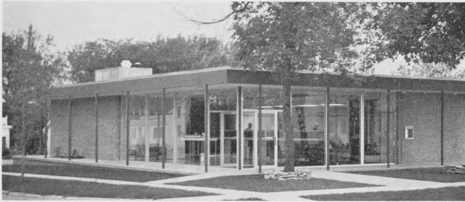
NEW BUILDING for American Sav. Bk., Tripoli.
