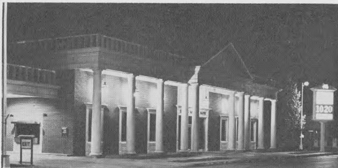
EXTERIOR and interior of new building for LeMars Savings Bank. More than 5,000 persons toured the new building at the formal opening recently, according to Gordon Mennen , presi-
