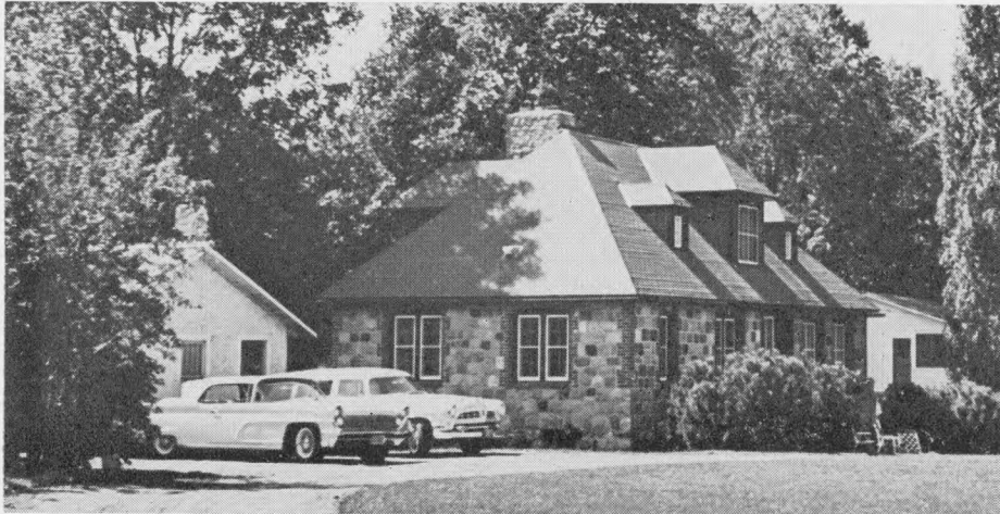
EMERGENCY shelter for First National Bank of Milaca.
