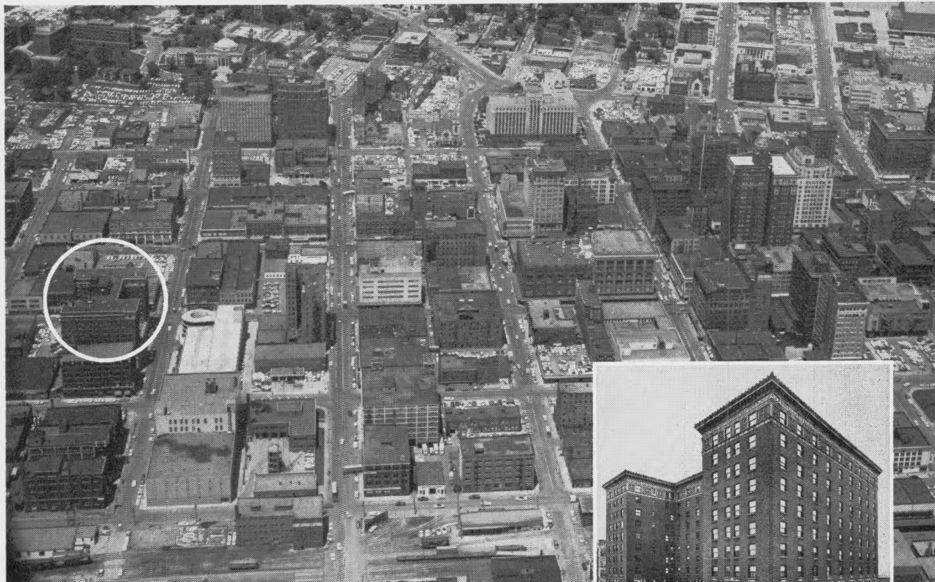
AERIAL VIEW DES MOINES, IOWA
