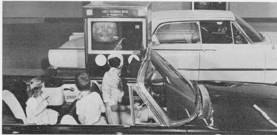
FIRST CUSTOMER stops at Mosler Autobank at the First National, Waukesha, Wis. Visible in the Autobank customer unit are the TV screen showing the teller in the bank and the TV camera which provides a picture of the customer for the bank teller.
