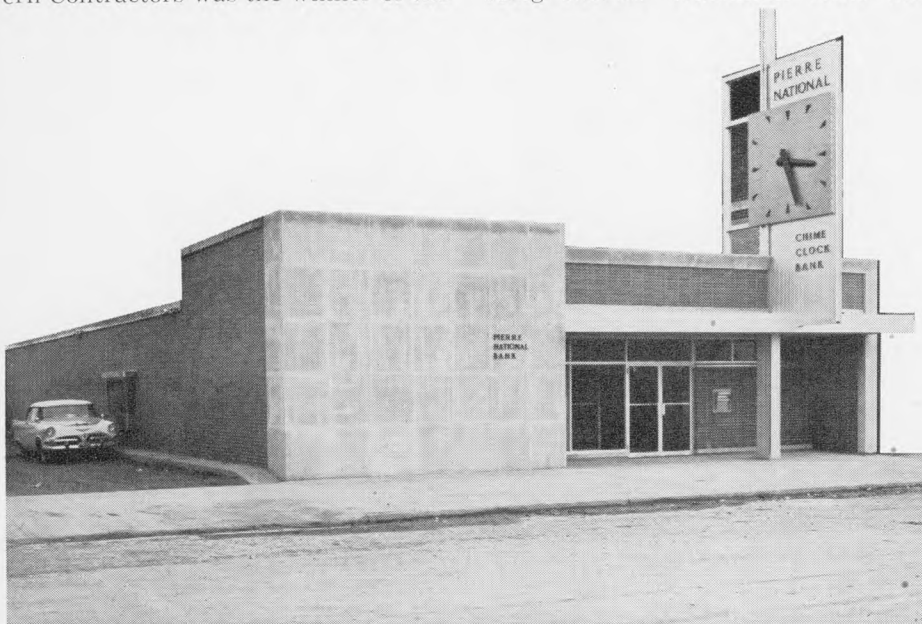
THE NEW CHIME CLOCK is one of the outstanding features of the new Pierre National Bank, and supplementing its telling of time with its eight-foot face is a set of musical chimes which play the same tune as did the bank's old clock. A final official count revealed that 5,700 persons attended the open house.
