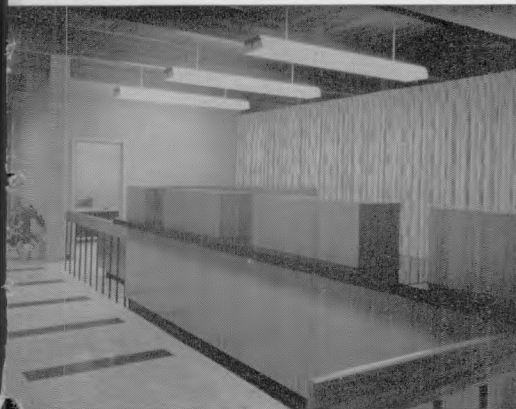
This neat, functional interior attracts business and speeds up service due to scientific planning of traffic flow. Another example of how Western Bank Contractors' knowledge and experience pay off in business-building efficiency.
