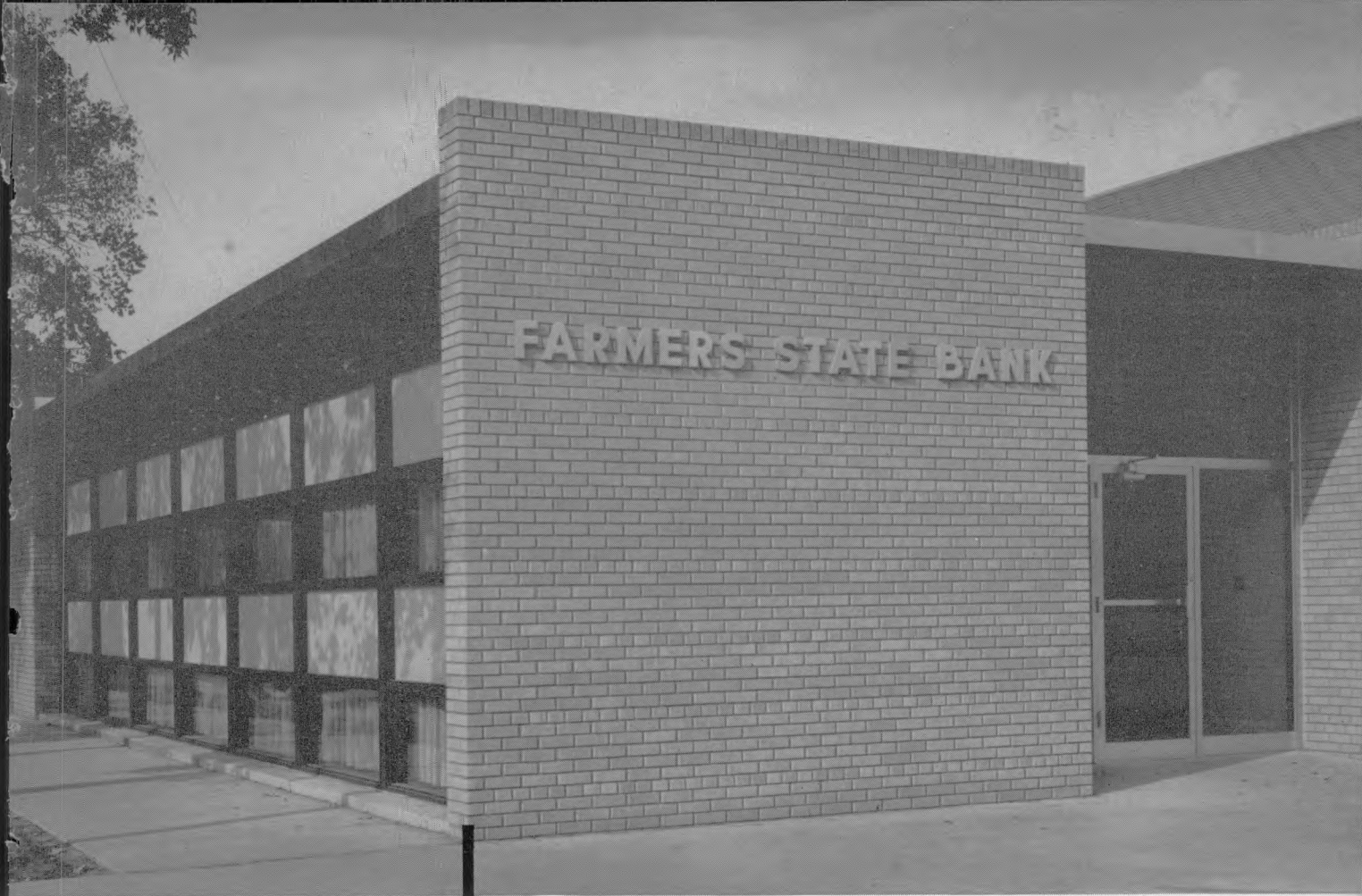
The new, modern-to-the-minute Farmers State Bank of Sargent, Nebraska, recently constructed by Western Bank Contractors, Inc., Kansas City, Missouri.
