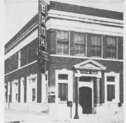
THE CITIZENS BANK OF CLOVIS, New Mexico, obtains peak efficiency with its National Unit Plan.
