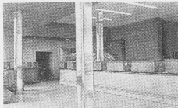
AFTER remodeling by JAEGER; Burlington Bank & Trust Co.
