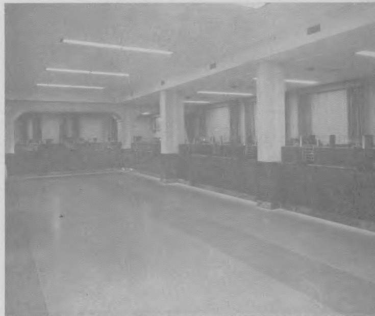
New quarters of the Millikin National Bank, Decatur, Illinois , as well as those of most Bank Building and Equipment Corporation jobs, are completely air conditioned. Drapes and venetian blinds lend cordial touch to back-counter areas. Teller counters are of the low sloping die front construction; wickets are decorative metal. Flooring is terrazzo. Low plate glass and metal railings separate portion of officers' section from main banking room.
