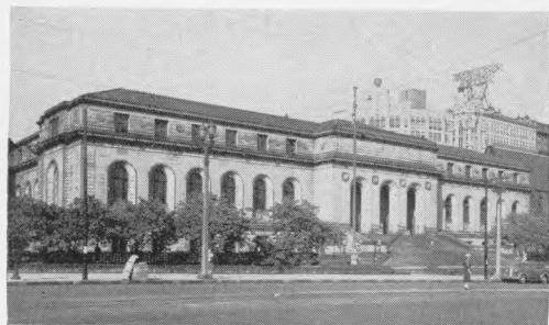
The Central Building of the St. Louis Public Library is part of the architectural group forming the Memorial Plaza. The Library contains approximately 960,000 volumes, has 22 branches, 104 sub-stations, and traveling libraries operated in connection with the public schools.
