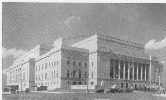
Henry Kiel Auditorium, facing Memorial Plaza in the heart of the downtown section of St. Louis, represents an investment of nearly $7,000,000 and is outstanding among convention halls in the country.
