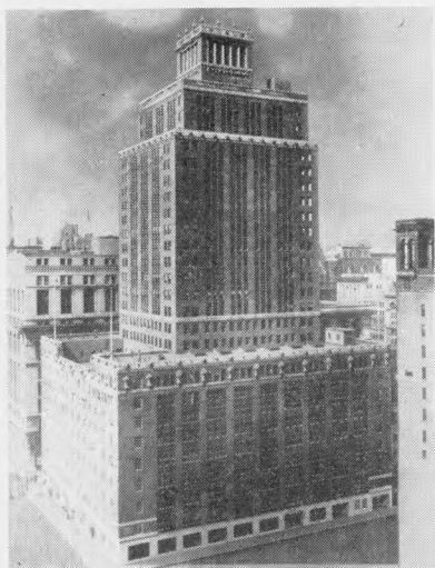
The Combustion Engineering Building at 12 East 36th Street, New York, N. Y., to which the American Bankers Association's national headquarters will move on or about December 1. The Association's offices will occupy the entire ninth floor.
