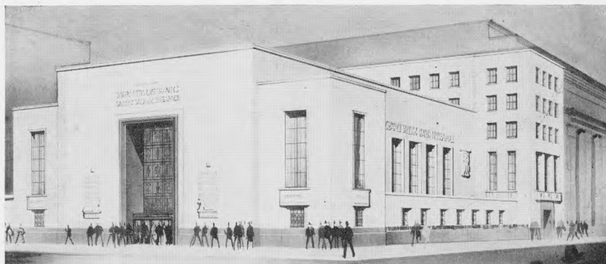
Here is the artist's conception of what the Farmers and Mechanics Savings Bank of Minneapolis will look like, which is now under construction in Minneapolis.
