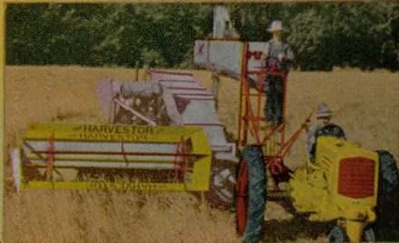
Harvester (8 ft.) with engine drive and MM "R" tractor harvesting wheat with real economy.
