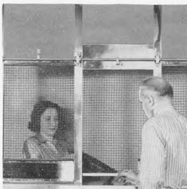
This is a view into the lobby from the opposite side of the wicket structure. The armor-steel shutters are pushed up out of sight and out of the way.
