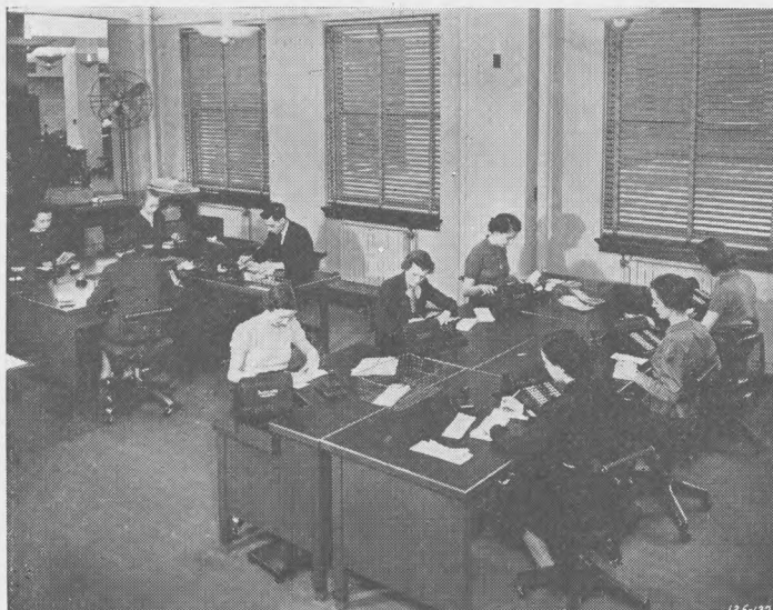
One of the highlights of the Northwestern National Bank and Trust Company's new proof department operation is their method of proving deposits. This group of electric duplex calculators, which accumulate individual totals and a grand total at the same time, makes it a fast, simple routine.
