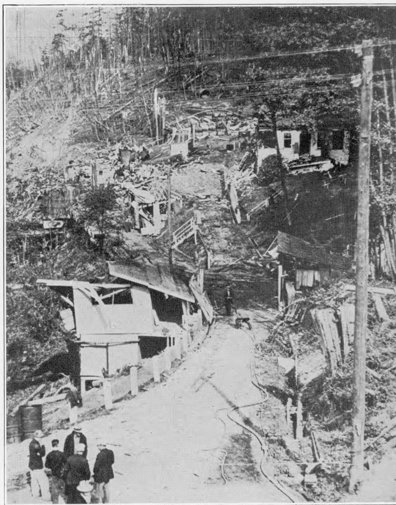
Fire insurance is not the sole coverage that is needed by most industrial concerns. The above shows the result of an explosion killing one person, injuring fifty others, and causing a half million dollars of property damage when the plant of the Puget Sound and Alaska Powder Company was wrecked by two explosions near Seattle. Photo, Wide World Studios
