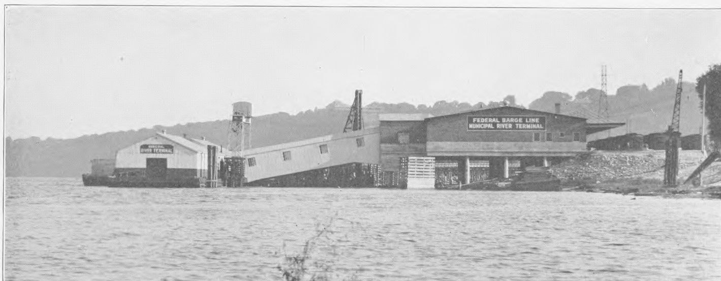
Dubuque's recently completed general cargo terminal, a part of the half-million dollar river terminal facilities at Dubuque
