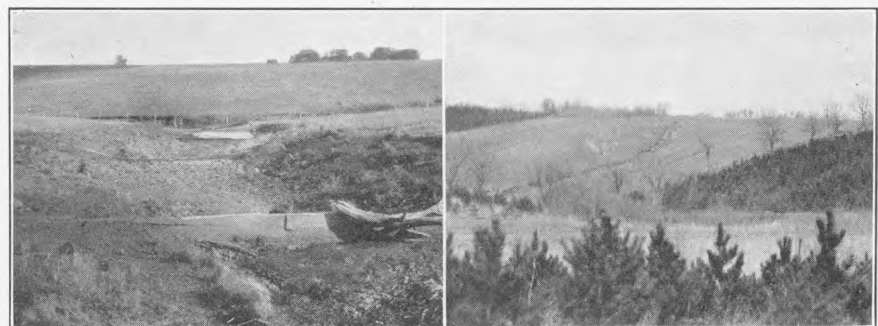
Dams properly constructed as shown on the left, will help prevent erosion and make it possible to farm the ditches. Some hillsides that are badly washed are suitable for reforestation. This picture at the right was taken on the Indian reservation near Tama, Iowa, and shows how trees may be grown successfully on land that otherwise is going to waste.
