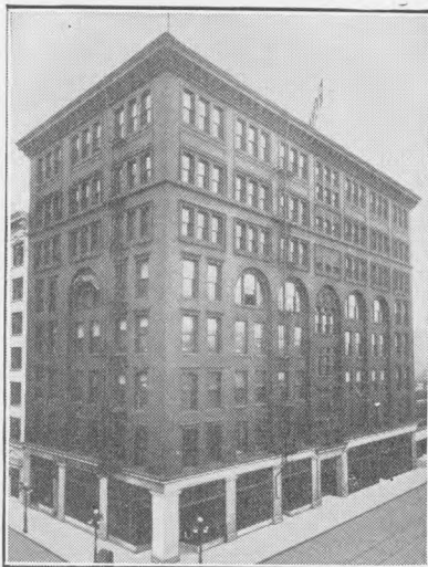
Royal Union Life Building, Cor. 7th and Grand Avenue, Des Moines, Iowa
